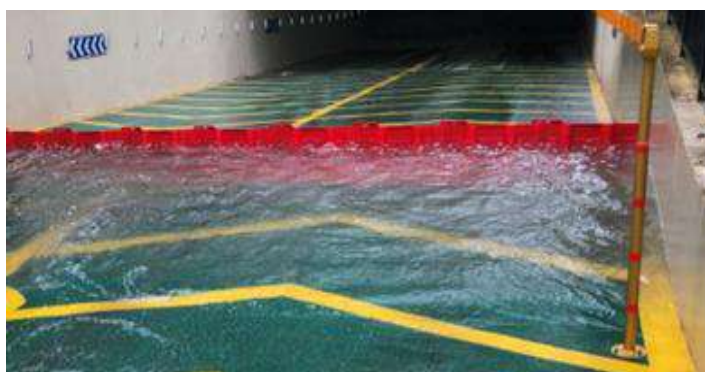
Foto 29. Barrera BOX de Lakeside Flood solutions
